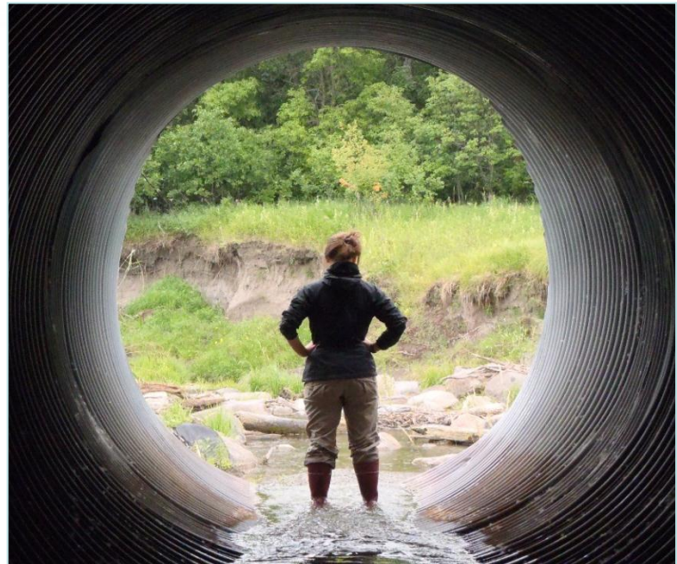
Masters student Noel Galuschik surveys bank erosion from a culvert in Manitoba. This field work is part of our Tobacco Creek research project profiled on page 2. Photo by Raea Gooding.
